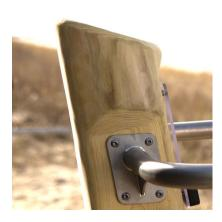
Construction made of Robinia - very durable acacia wood with a diameter of  $\sim 22$  cm without sharp edges, resistant to weather conditions,
