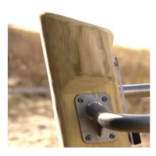
Construction made of Robinia - very durable acacia wood with a diameter of ~ 18 cm
