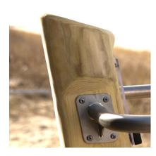
Construction made of Robinia - very durable acacia wood with a diameter of  $\sim 18~\text{cm}$  without sharp edges, resistant to weather conditions.
